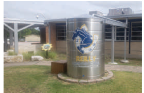
Reilly Elementary School in central Austin won a national competition for its rain capturing system
